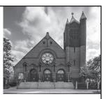
The main capital improvement project completed last year was the repair and tuck pointing of the St. Gabriel bell tower. Further tuck pointing will be required for the lower portion and for the church in the near future. In addition, we will begin considering replacing the carpet in the church and perhaps the kneelers. Spacing out the pews by a few more inches might also be worth considering.
